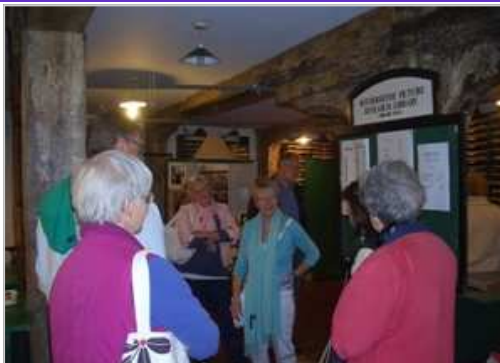
Roof beams made from ship's timbers
